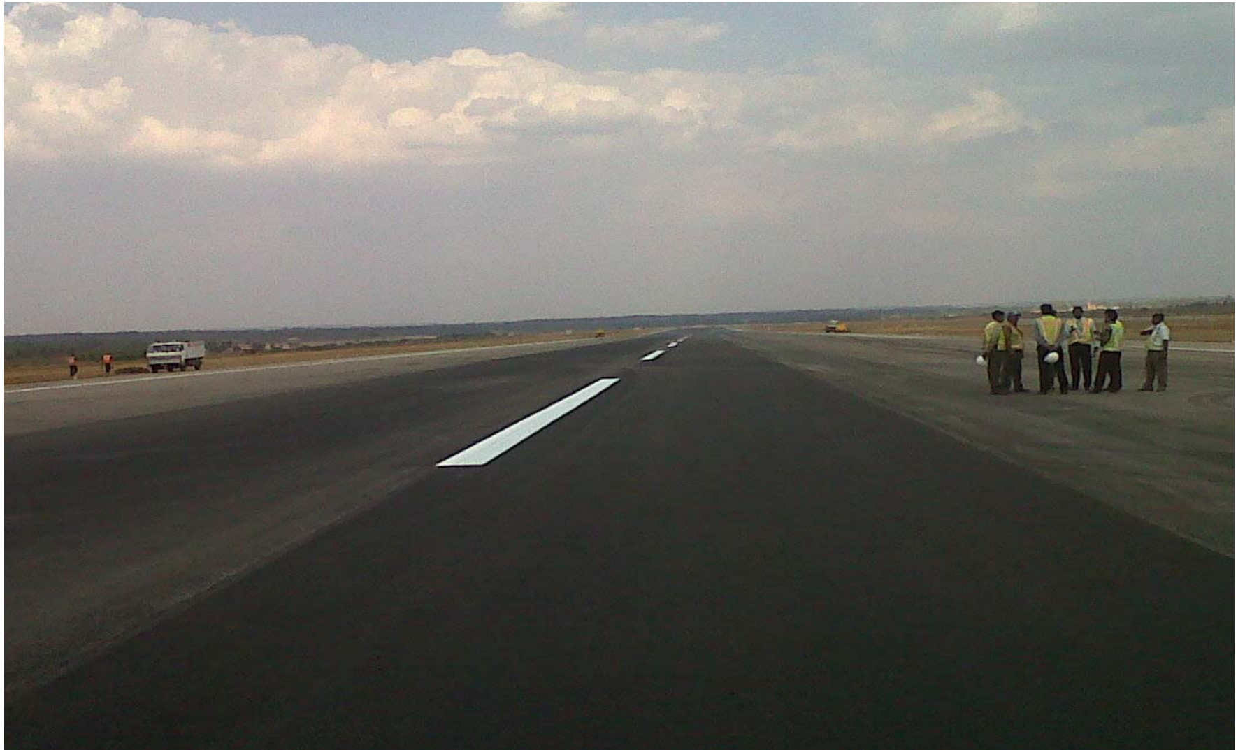
Inspection of Relayed runway surface by RST
